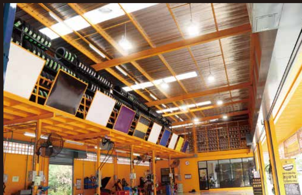
Lights inside the pit of B-Quik, Thailand
